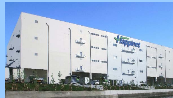
Happinet Second Logistics Center-East (operated February 2006)
