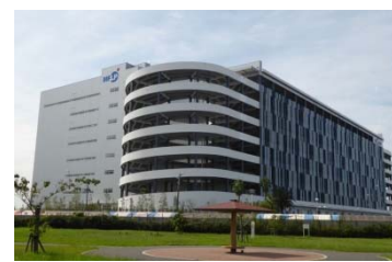
Second Logistics Center-East Japan
