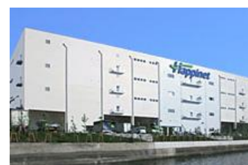
Second Logistics Center-East Japan
