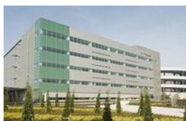
Logistics Center-West Japan
