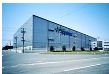
Logistics Center-East Japan
