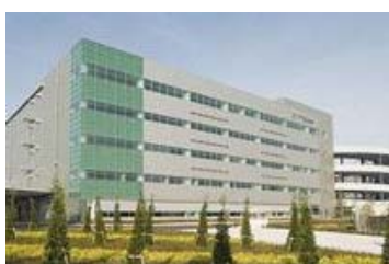
Logistics Center-West Japan
