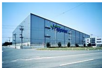
Logistics Center-East Japan
