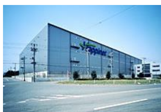
Logistics Center-East Japan
