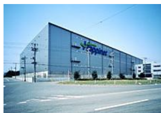
Logistics Center-East Japan
